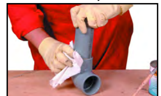
Wiping away excess cement
