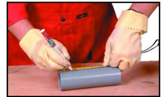
Marking the pipe end
