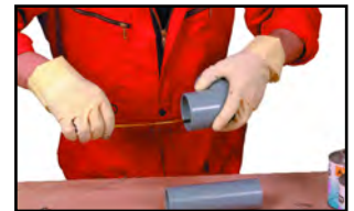
Measuring the insertion depth
