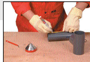
Marking the pipe end
