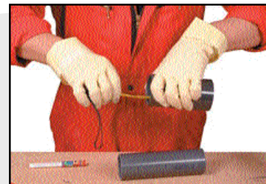
Measuring the insertion depth
