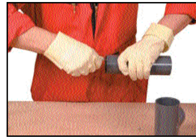
Removing the internal burr
