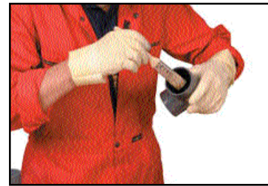
Brush applying cement to the fitting
