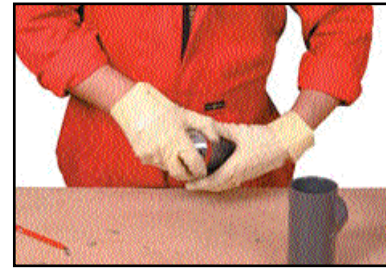
Chamfering the pipe
