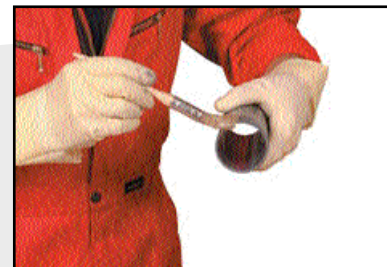
Brush applying cement to the pipe
